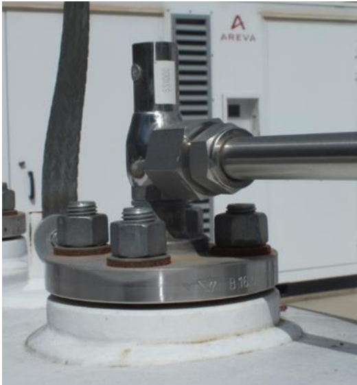
Figure 68 : Areva backup System (pressure release device detail) ©AREVA/ENSOSP 2015
