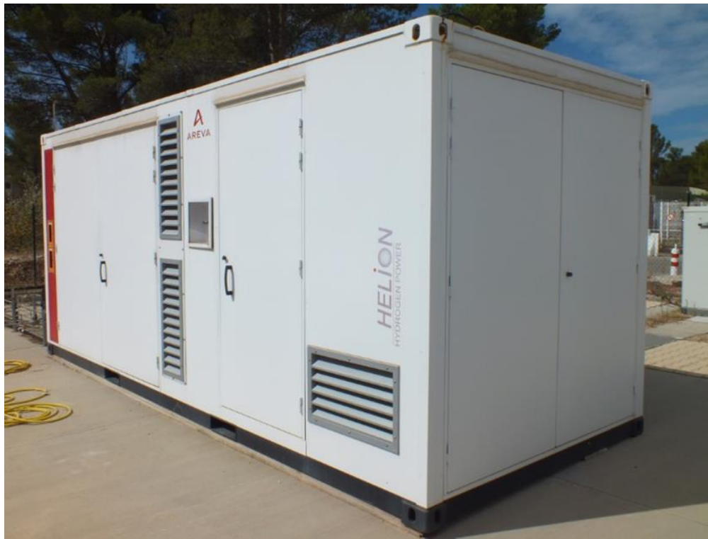
Figure 65 : Areva backup System (fuel cell compartment) ©AREVA/ENSOSP 2015
